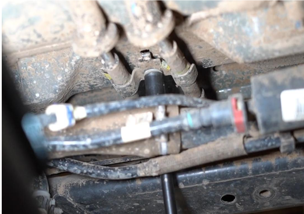
Figure 30: Emergency cable bracket tightened
